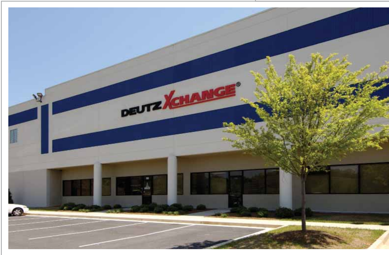
DEUTZ Xchange production facility
