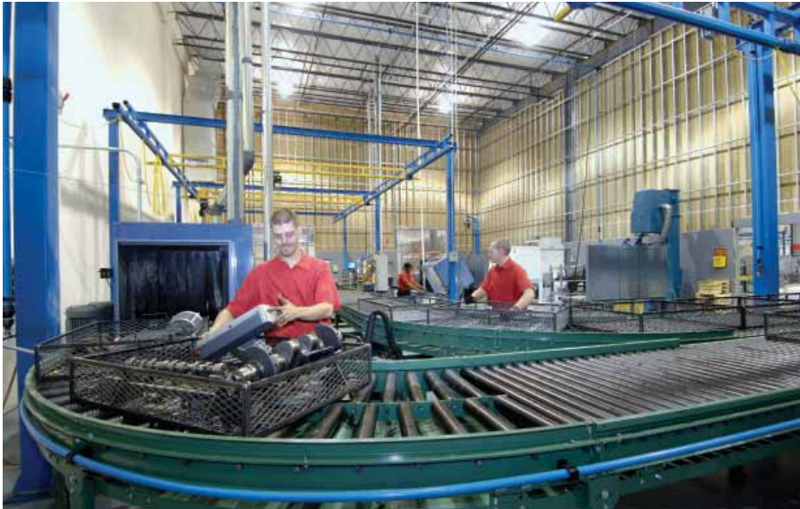
AREA 2: High Temperature parts wash
